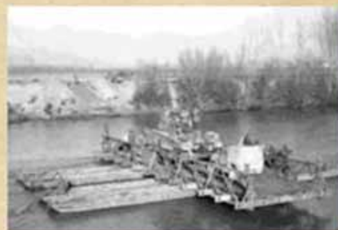
The first tanks cross the Garigliano
